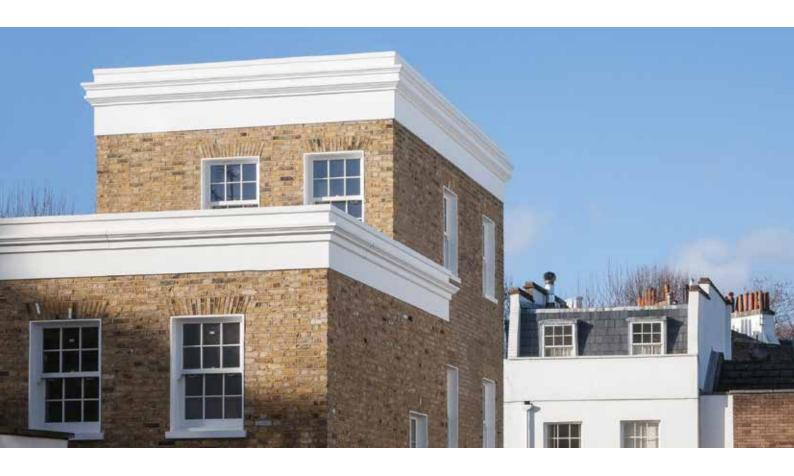
The original cornice and frieze to this period London townhouse had crumbled away. The replacement mouldings matching the original detail were supplied and installed by Stevensons of Norwich with a paint finish to be applied afterwards.
